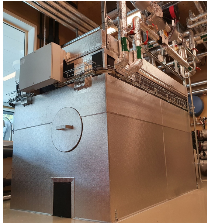
Fig. 1. A photo of the latent heat storage unit in the zero-emission building.
