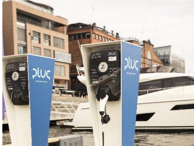
Figure 3 Maritime charging station with Zaptec charger and type 2 connector in Oslo. Image: Plug
