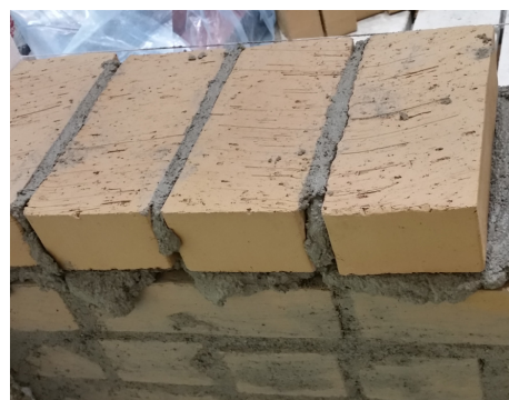
Figure 2. Close-up of bricks during brick laying.
