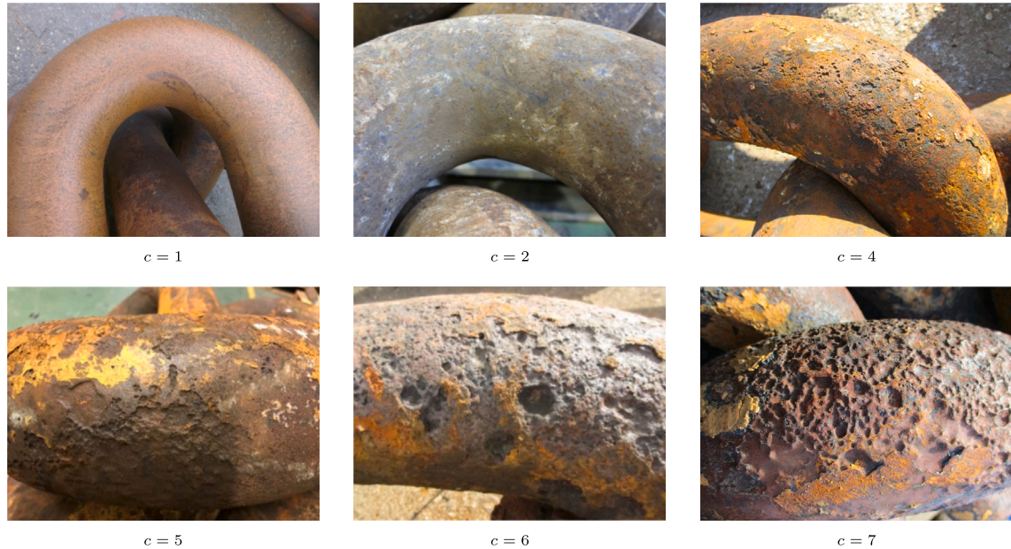
Fig. 1. Examples of corrosion grades (c). None of the used chain samples in the database were graded with c = 3 .
