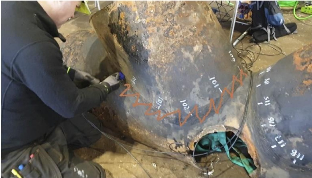
Figure 2. The recording of the actual dataset was performed onshore. The probe was moved along a welding in a zigzag movement, as indicated by the orange painted line.
