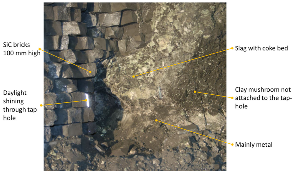
Fig. 8. The coke bed in front of the tap hole, with a clay mushroom on the inside of the coke bed. Reprinted with permission. 18
