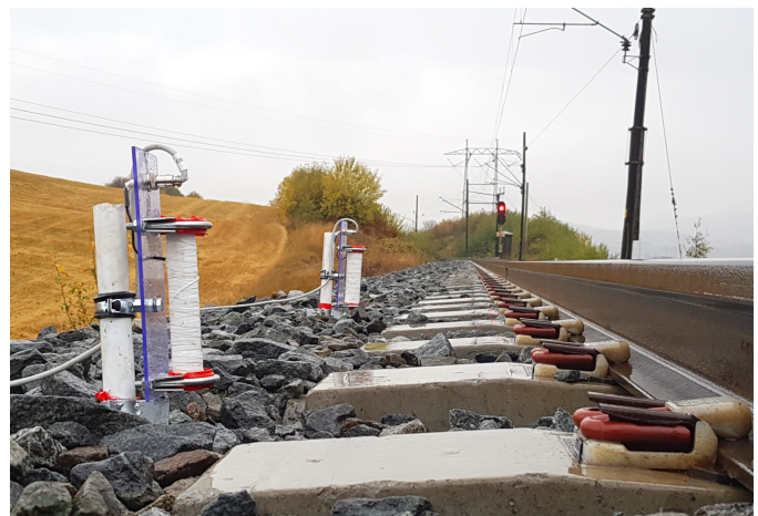
Fig. 11: The coils were placed a distance of 0.5 m from the nearest rail, here shown in the sloped location.
