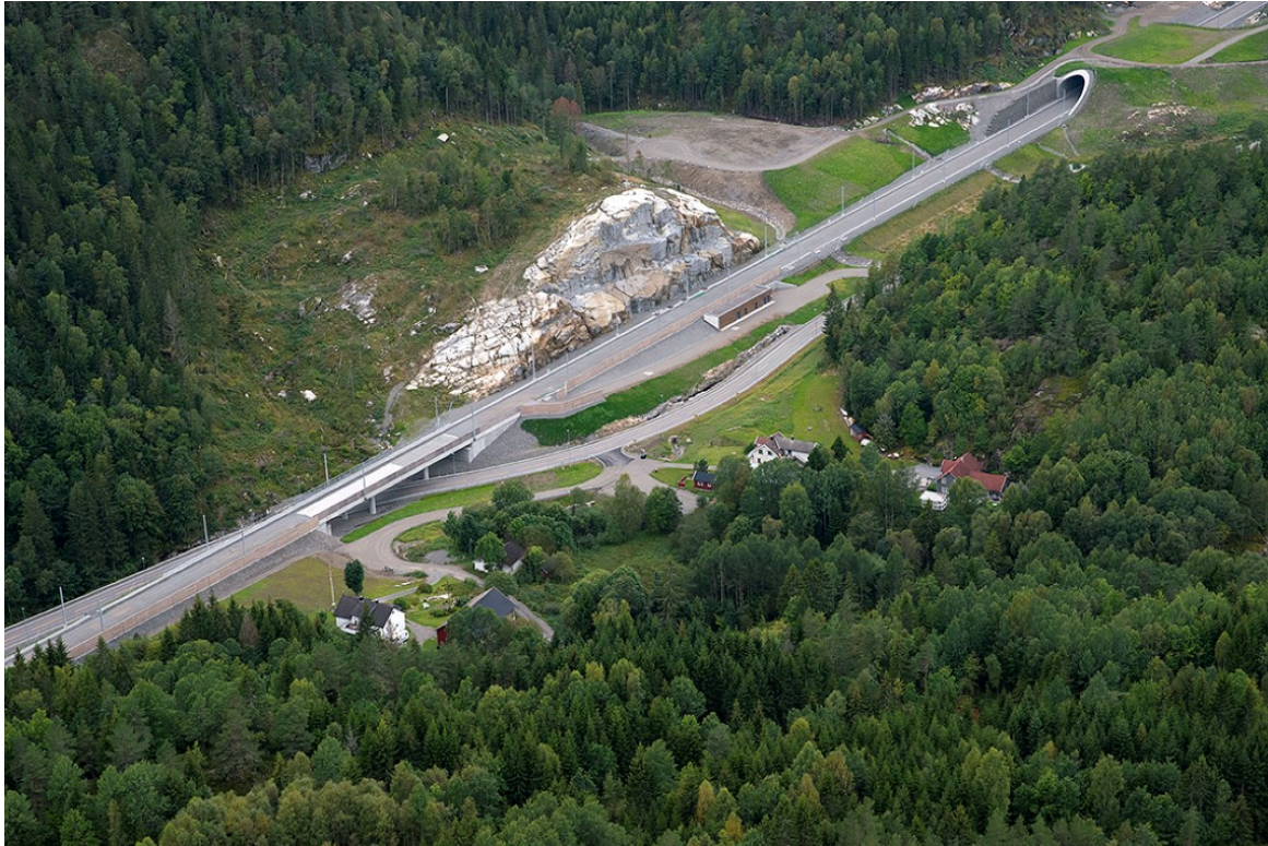
Figure 43: Entrance of one of the tunnels [90].
