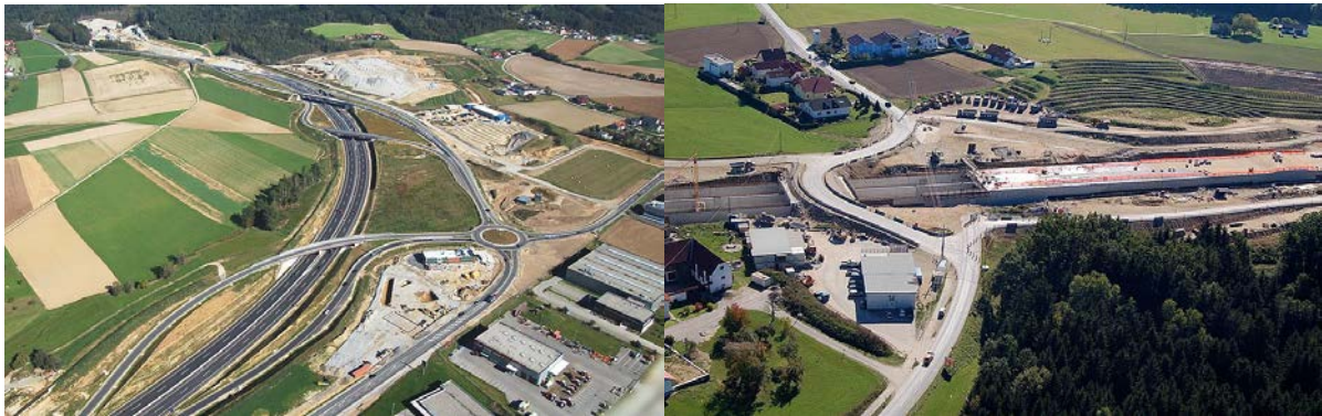
Figure 39 Pictures of the construction [87].
