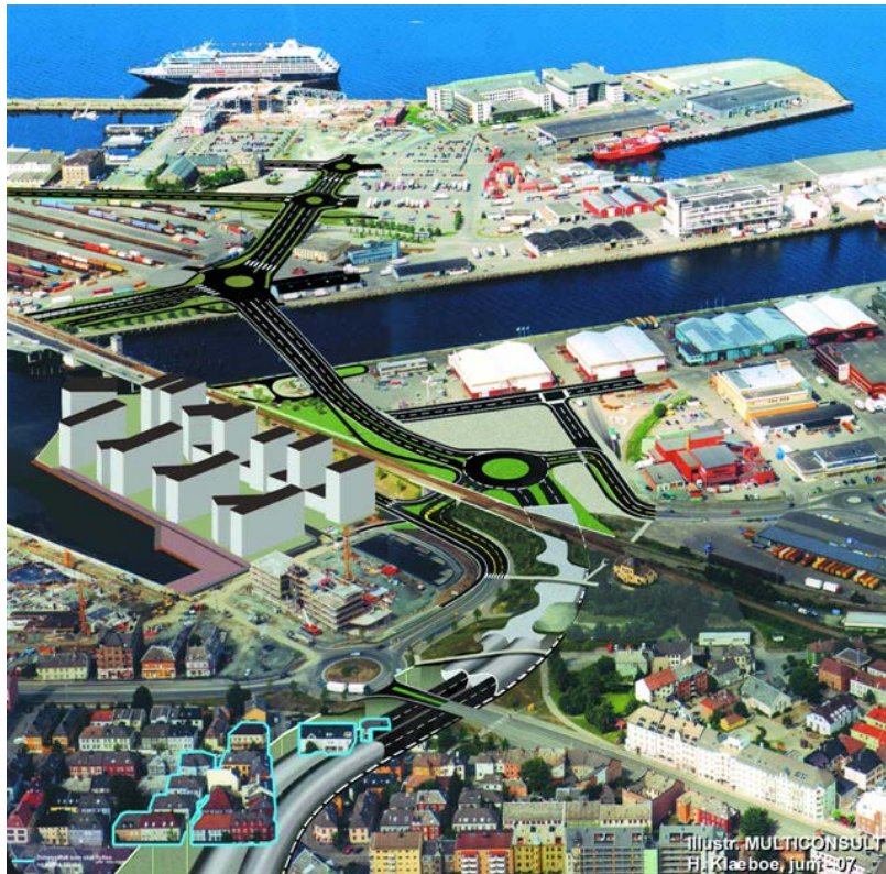
Figure 38: Overview of the Strindheim tunnel (Statens Vegvesen).
