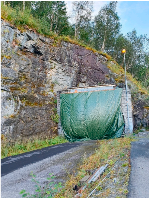
Fig. 3. Entrance to the tunnel covered by a tarpaulin to avoid daylight coming in. Photo: Carl Södersten, SINTEF.
