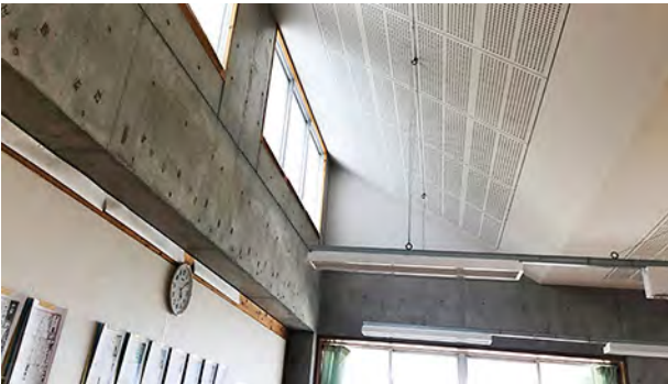
Figure 3. Vertical ceiling windows
