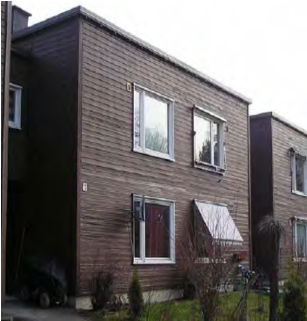
Figure 1 The demo building prior to refurbishment.
