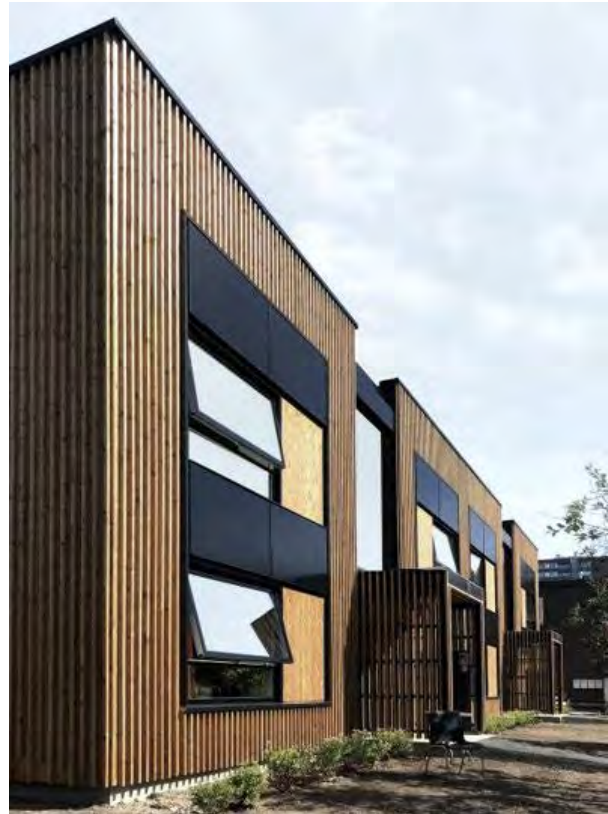
Figure 2 The demo building after refurbishment.
