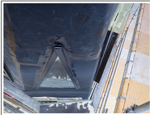
Figure 2. Tape used to seal the wind barrier around a window.
