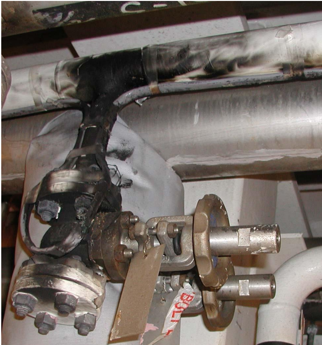
Figure 3: Burnt-out cable, BSX3-2, on a firewater pipe at Snorre B. A loop of the cable is laid around a flange. The point of failure on the cable seem to be situated close to the edge of the flange. An earth fault alarm led to detection of the failure.
