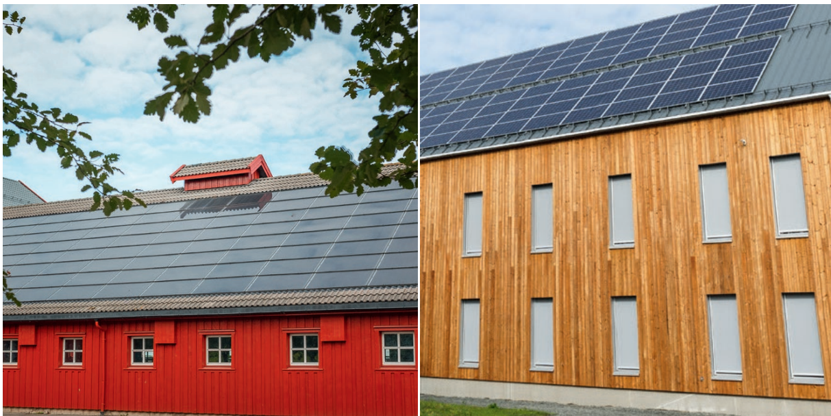
Figure 59. Left: PV system on the Building Z (calf barn). Right: PV system on the Building I (dormitory). Photos courtesy of Mære Landsbrukskole.
