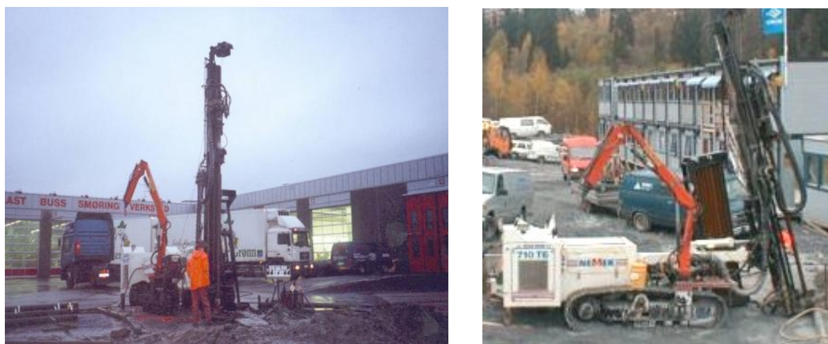
Figure 4.8 Drilling of energy wells by pneumatically driven rigs (Båsum, 2004).
