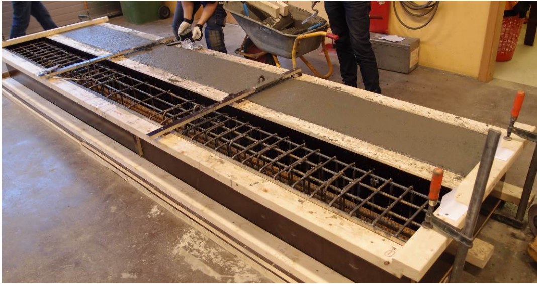
Figure 2.3: Beam 1A casted and beam 1B prepared for casting
