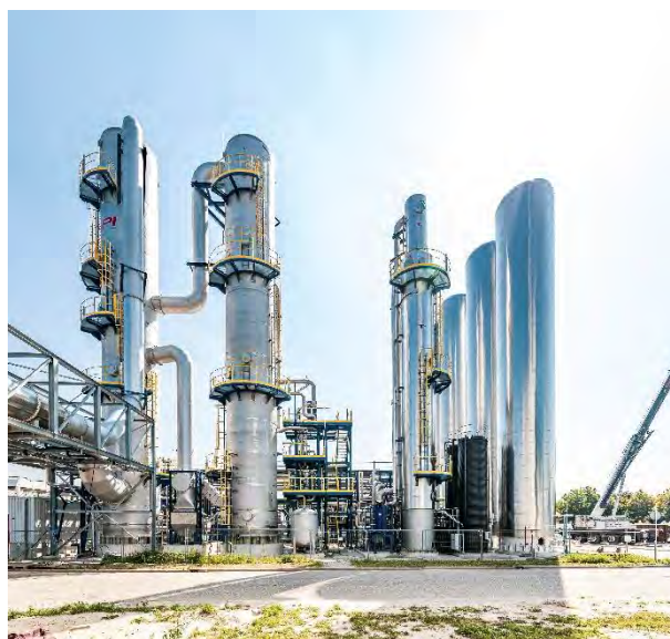
Figure 1, the commercial AVR CO 2 capture plant in Duiven, The Netherlands [2].
