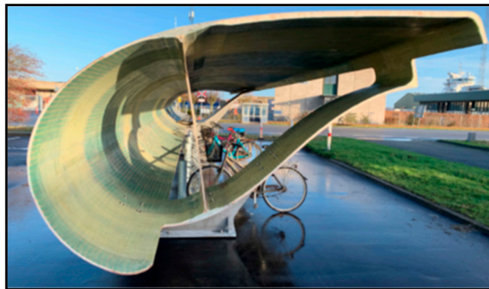
Figure 7. Examples for rotor blade repurposing: bike shed (source: Re-Wind and Port of Aalborg, Denmark, Wind Europe Report 2020), reproduced with permission of WindEurope [13].
