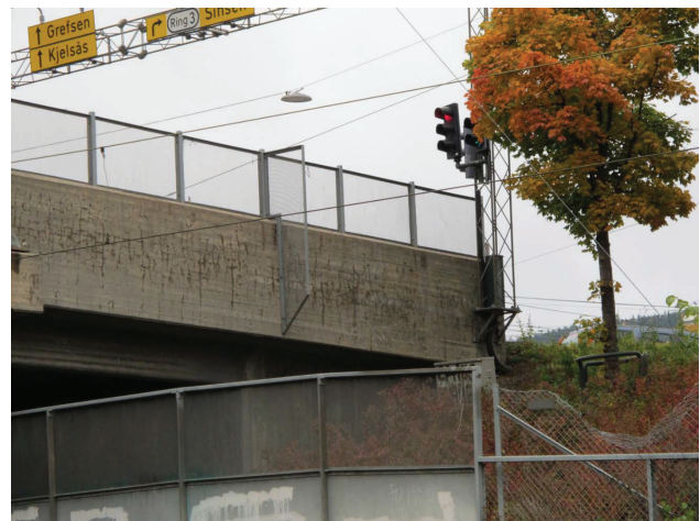
Figure 2 The Storo bridge, southern side [4]
