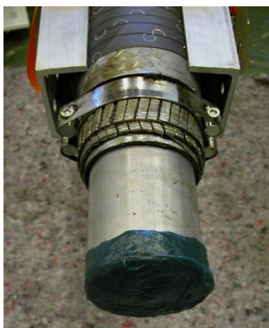
Figure 3. Cable end with the outer layers stepwise removed and cleaned. A polyester padding temporarily covers the end surface of the insulation and the conductor, preventing air ingress.
