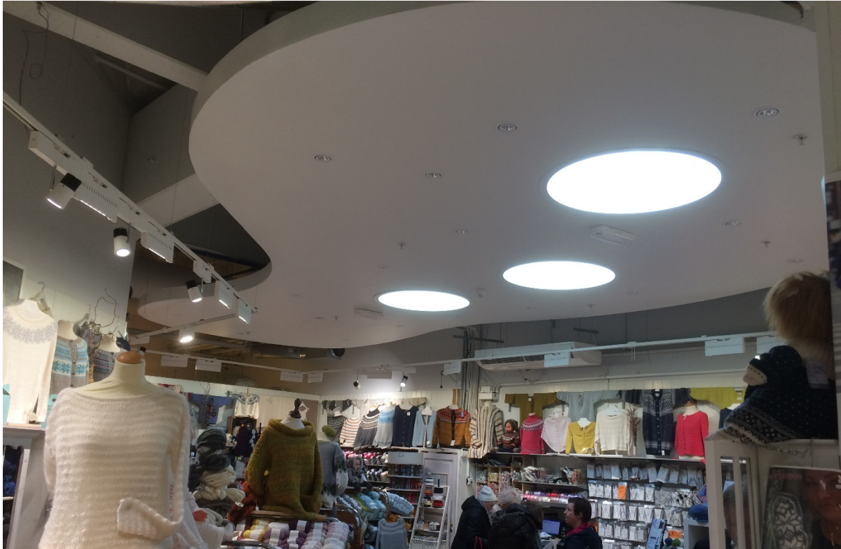
Figure 32 Shopping centre in Trondheim, Norway. Three light pipes have been mounted in one shop.
