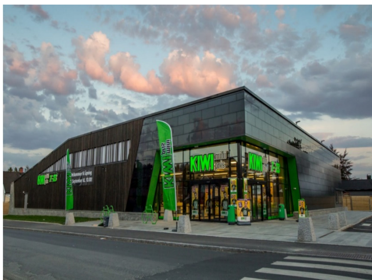
Figure 14 KIWI Dalgård in Trondheim. Parts of the façade is covered with building integrated solar cells [29].
