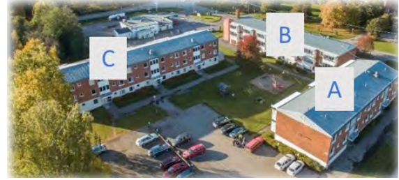
Figure 2 Bird view of the case building cluster located in Ludvika, Sweden
