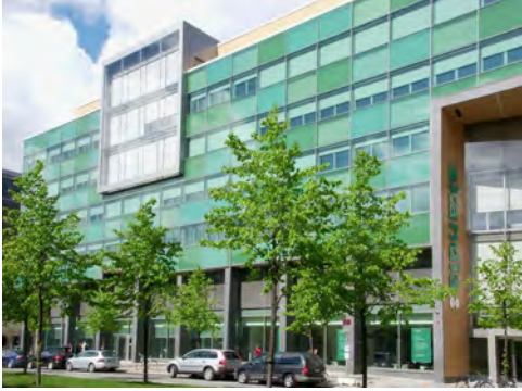
Figure 1: Gångaren 11, double skin façade building envelope
