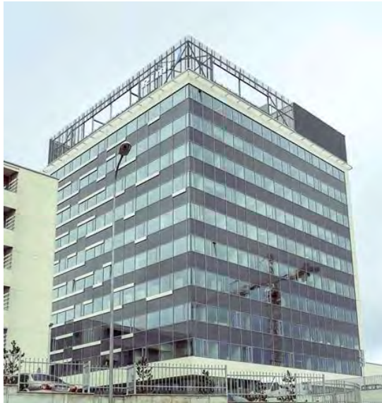
Figure 1 Photo of the building
