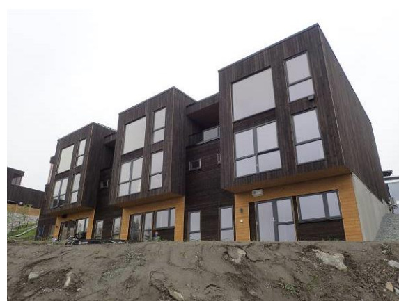
Fig. 6. The building that is part of the pilot project in Malvik. (Photo: Tore Kvande)
