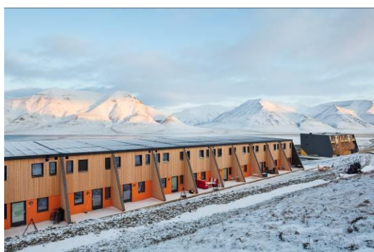
Fig. 2. One of the buildings that are part the pilot project in Longyearbyen. (Photo: Trond A. Isaksen)
