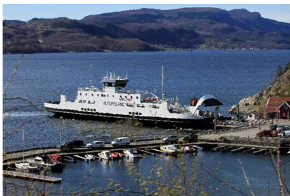
Figure 13: Ferry port across the municipal border, where hydrogen ferry will land from 2021 (photo: Andreas Askildsen/Stavanger Aftenblad).
