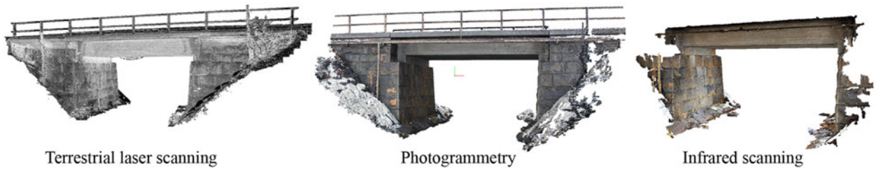
Figure 9. 3D models of Pahtajokk bridge—differences in level of detail between the tested methods.
