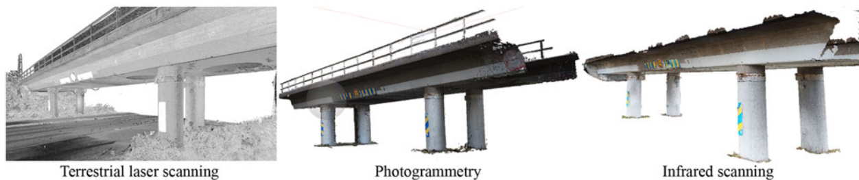
Figure 10. 3D models of Kallkällevägen bridge—differences in level of detail between the tested methods.
