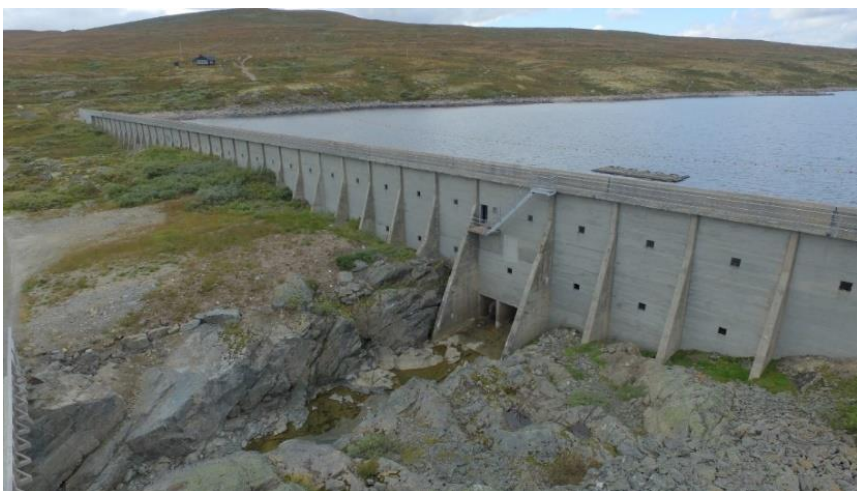
Figure 1. Aerial view of Kalhovd Dam.
