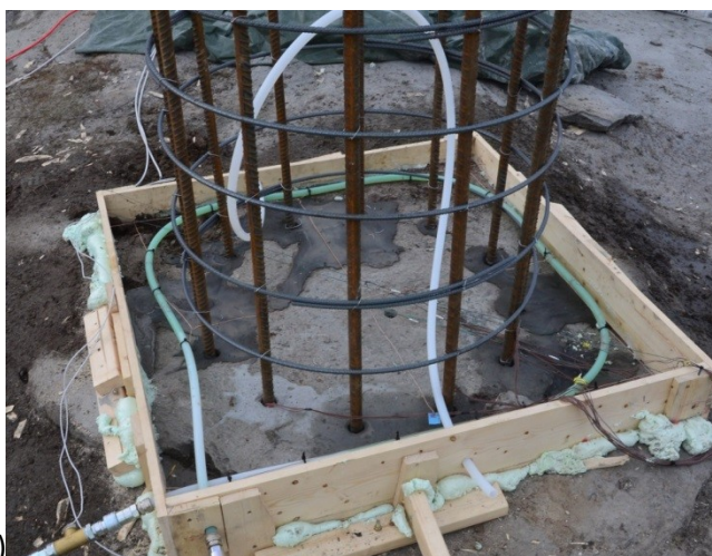
Fig. 4 (a) PERT Heat loop in the footing prior to casting, and (b) insulated footing during curing.
