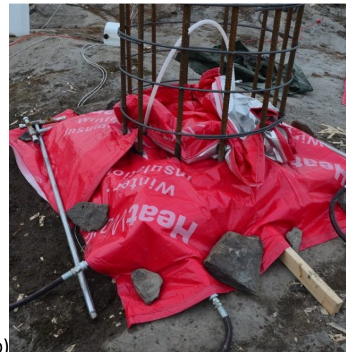
Fig. 4 (a) PERT Heat loop in the footing prior to casting, and (b) insulated footing during curing.
