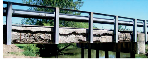
Figure 16. The Paint Creek Bridge (Stillings 2012).
