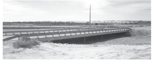
Figure 29. The Baandee Bridge (Pressley et al. 2004).
