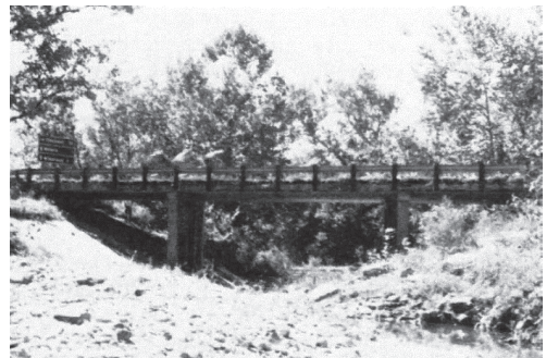
Figure 25. The Batavia Bridge (Aktan et al. 1992).
