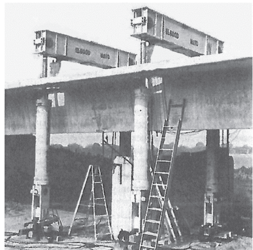
Figure 8. The loading of Pennsylvania State University Bridge (McClure & West 1984).
