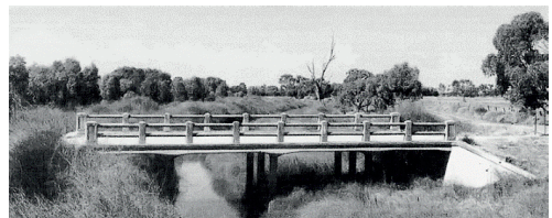
Figure 28. The Barr Creek Bridge (Haritos et al. 2000).
