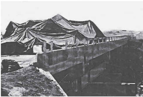
Figure 10. The Niobrara Bridge (Shekar et al. 1993).
