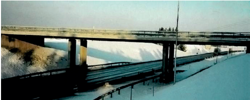
Figure 26. The Smedstua Bridge (Statens Vegvesen 1998).
