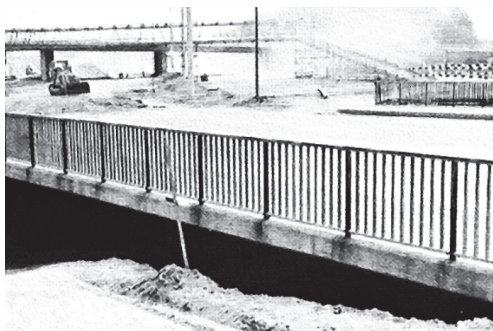
Figure 19. The Glatt Bridge 2 (Weder 1977).
