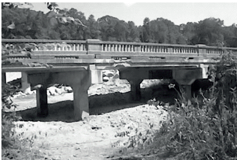
Figure 11. The Lennox Branch Bridge (Alkhrdaji et al. 1999).
