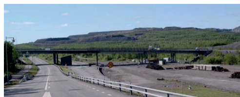
Figure 32. The Kiruna Bridge (Image by Niklas Bagge).
