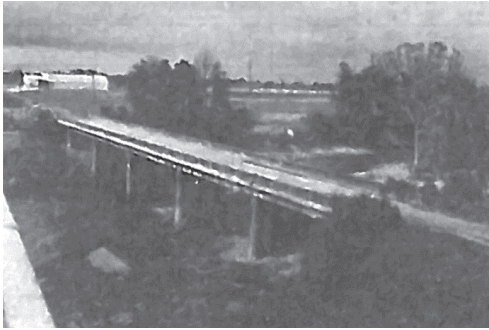
Figure 7. The Elk River Bridge (Burdette & Goodpasture 1973).
