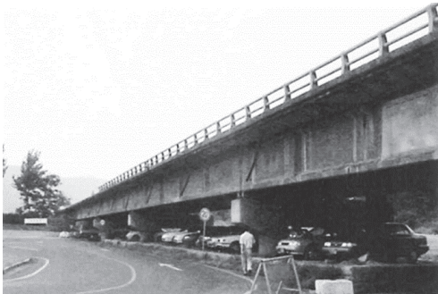
Figure 12. The Seoul-Pusan Highway Bridge (Oh et al. 2002).
