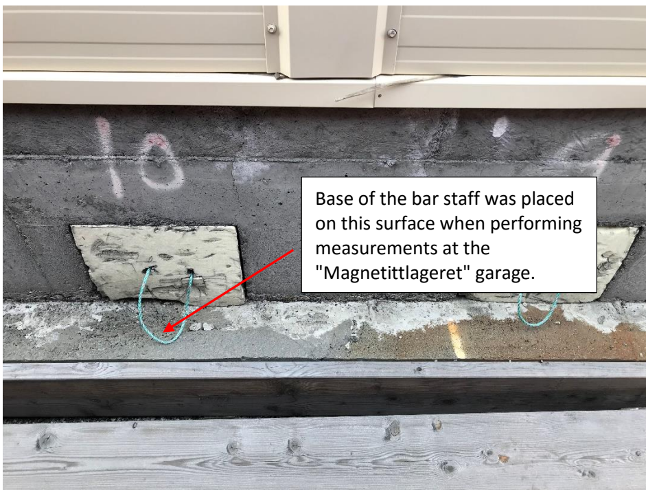
Figure 2. Measurement at the "Magnetittlageret" garage.
