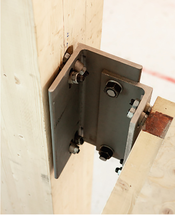
Fig. 8. Picture of the connector installed between the floor element and the column (photo: SINTEF/A.- L. Bakken).
