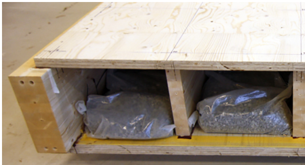
Fig. 6. Element cavity with the gravel bags.
