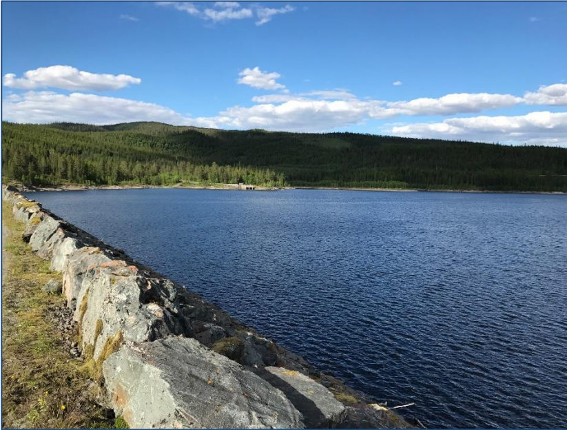
Figure 8.3. Shoreline protection, in this case due to hydropower regulation, changes the hydromorphological conditions of a lake (Photo: Tor Haakon Bakken).
