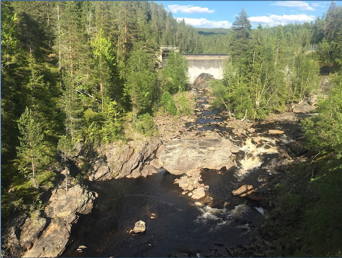
Figure 7.3. A weir can act as a barrier to upstream and downstream migration (Photo: Tor Haakon Bakken).
