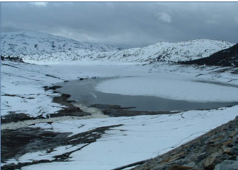
Figure 3.18. Reservoir drawdowns can cause large dewatered areas and block the access to tributaries (reduce connectivity) (Photo: Atle Harby).
