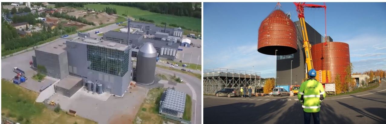
Figure 6: Eidsiva Bioenergi's Trehjørningen facilities in Hamar (NO) – Photo: Eidsiva Bioenergi AS.
