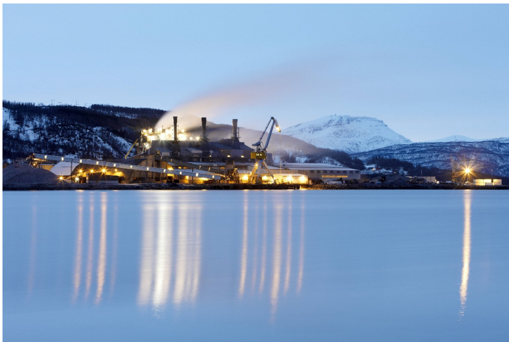
Figure 7: Finnfjord facilities in Finnsnes (NO) – Photo: MAN Energy Solutions.
