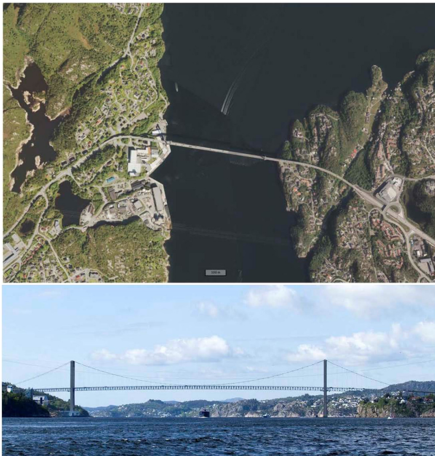
Figure 12: An overview of the Sotra bridge crossing
