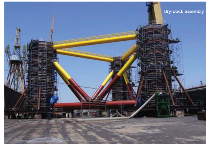
Columns moved to Dry-dock
