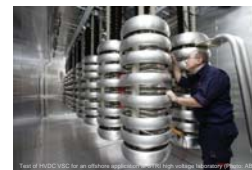
Test of HVDC VSC for an offshore application at the high voltage laboratory of STRI.
