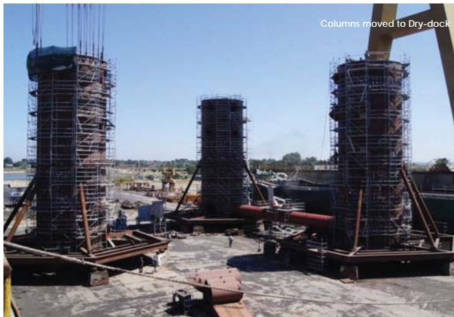
Pre-assembly of the columns outside the Dry-dock in Setúbal
