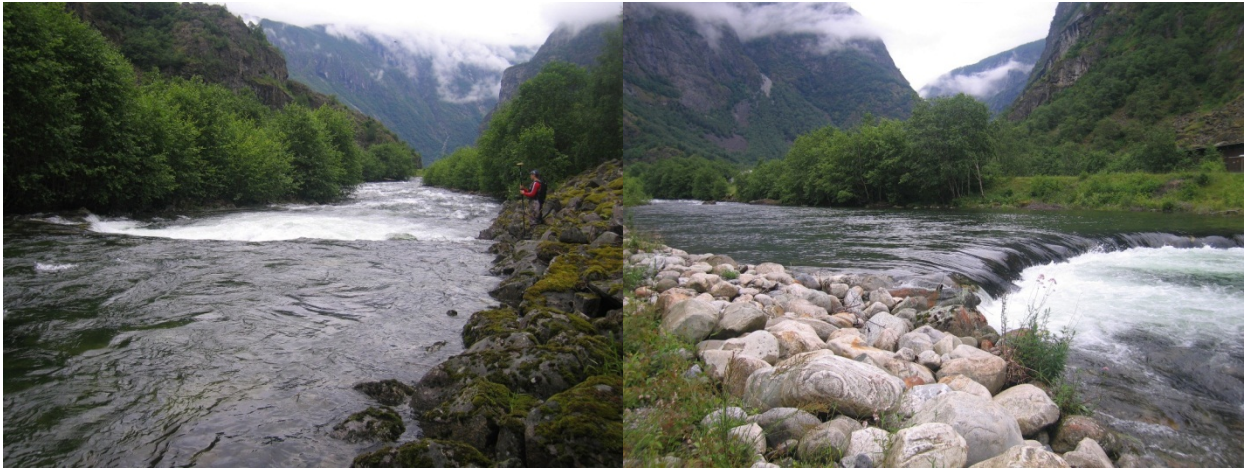
Figure 4.5 Artificial weirs and pools in Vassbydelvi at high flow around 16 \text{ m}^3/\text{s} .
