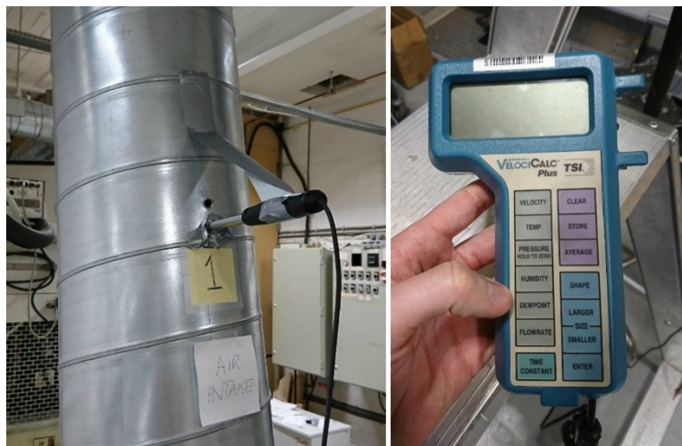
Figure 17 Picture of the lab setup (left) with the VelociCalc 9565-P mounted in the centre of the duct and picture of the VelociCalc 8388 (right).
