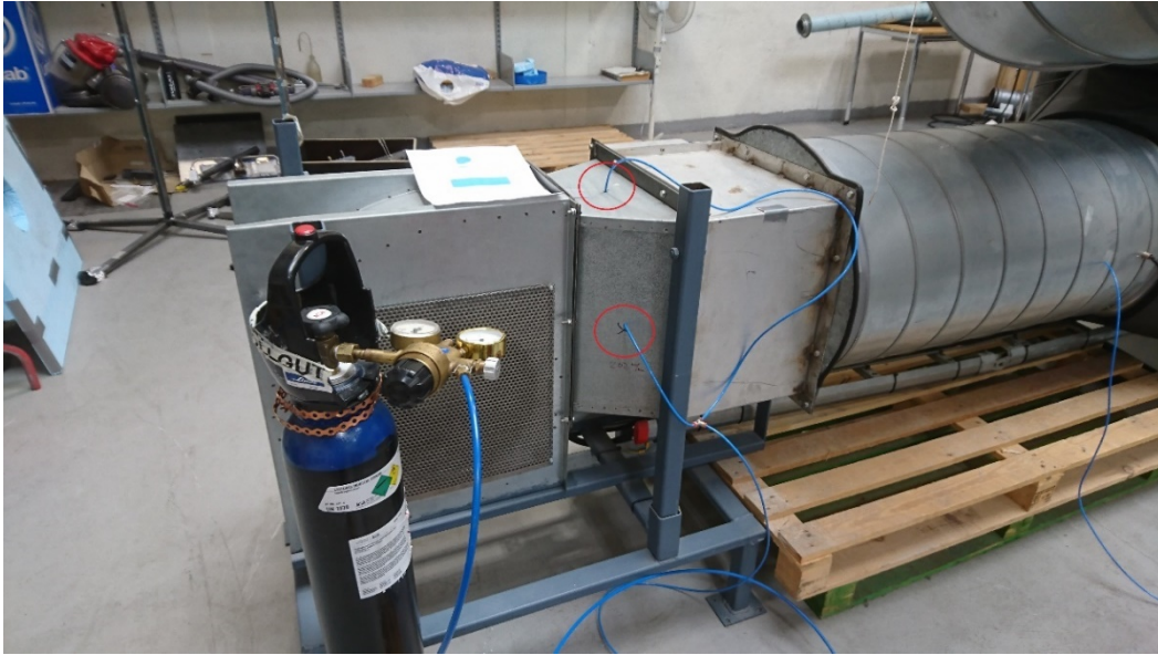
Figure 25 Picture of the duct where the tracer gas is released. Two tubes with multiple holes are inserted perpendicular to the duct as marked with red circles.
