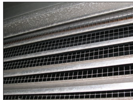
Photo 4: Closeup of metal grid and blinds from Photo 2 .
