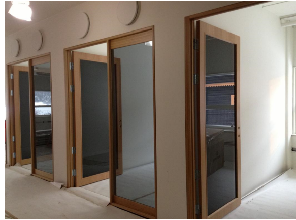
Figure 2.15 Interior office fronts with reused glass facade panels. Photo: Skanska.
