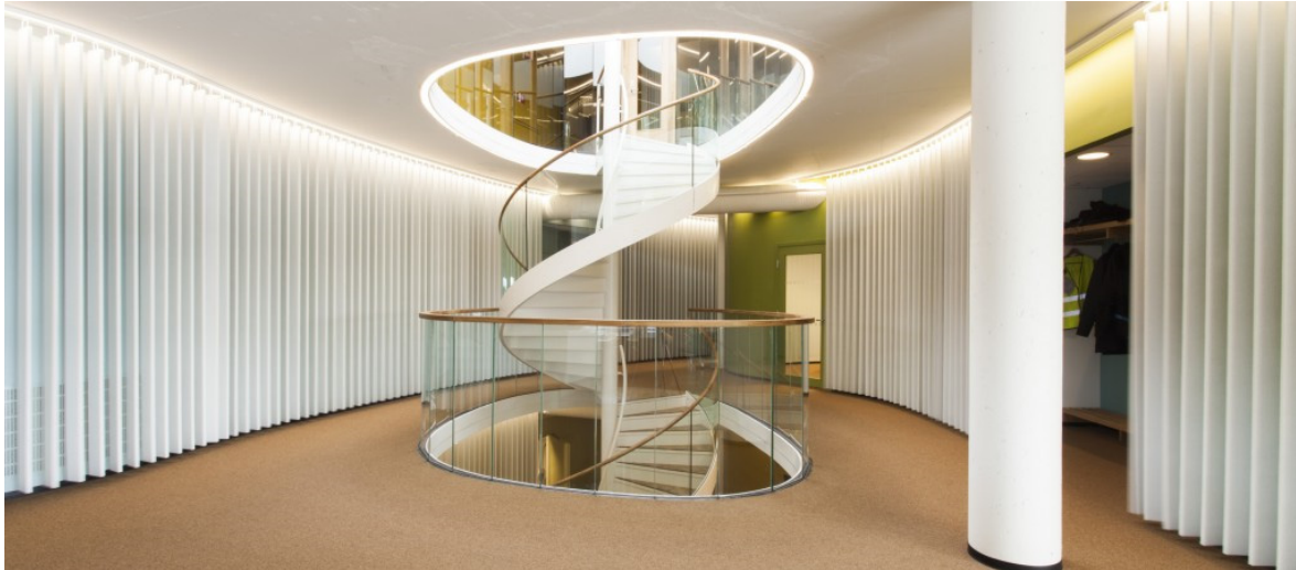
Figure 3.2 Picture showing exposed thermal mass in ceiling, vertical acoustic baffles on interior walls, and the central stairway that functions as a return air duct. A supply air diffuser is barely visible in the lower left corner of the picture. Photo: Chris Aadland / Asplan Viak.
