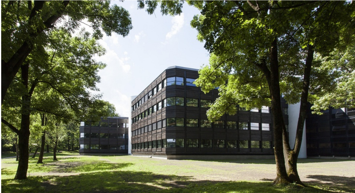
Figure 1.2 Building after renovation (right). Photo: Chris Aadland / Asplan Viak.
