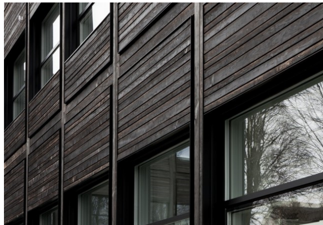
Figure 2.17 Charred wood in the façade. Photo: Skanska.
