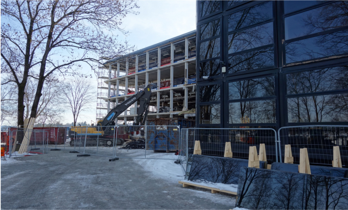
Figure 8.4 The Construction process at Powerhouse Kjørbo. Photo: Snøhetta
