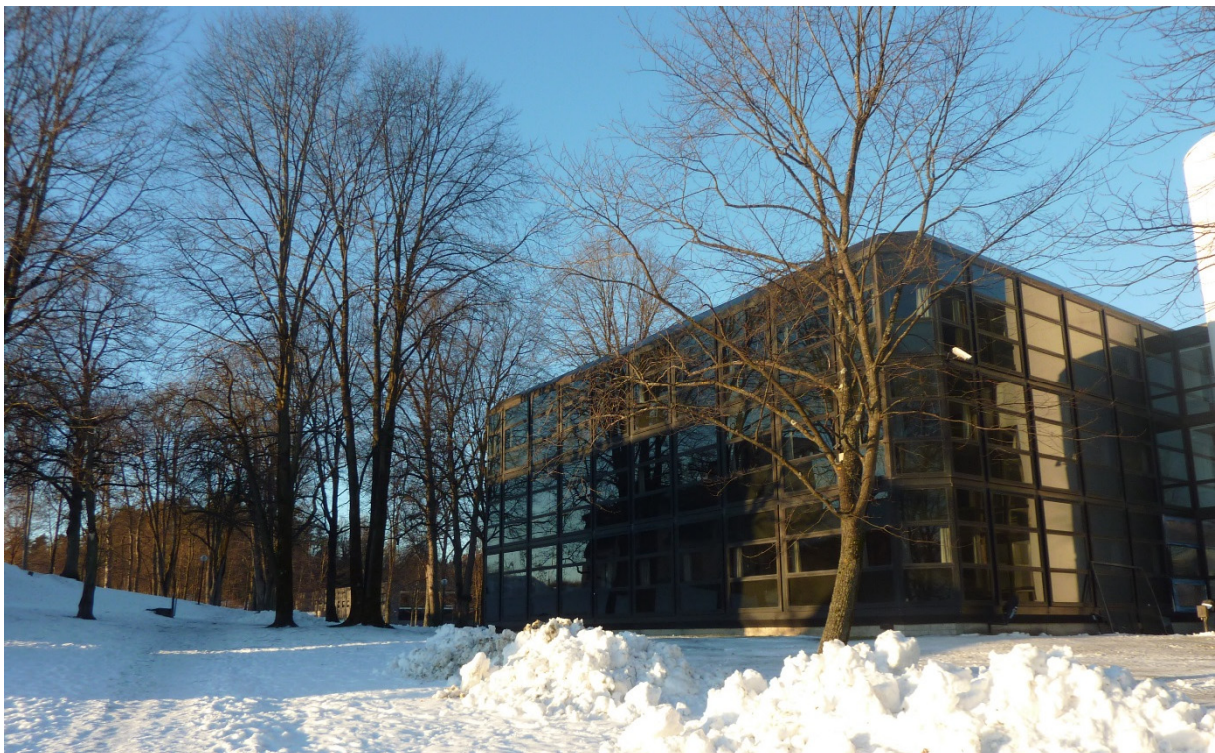
Figure 1.1 Building before renovation. Photo: Skanska.
