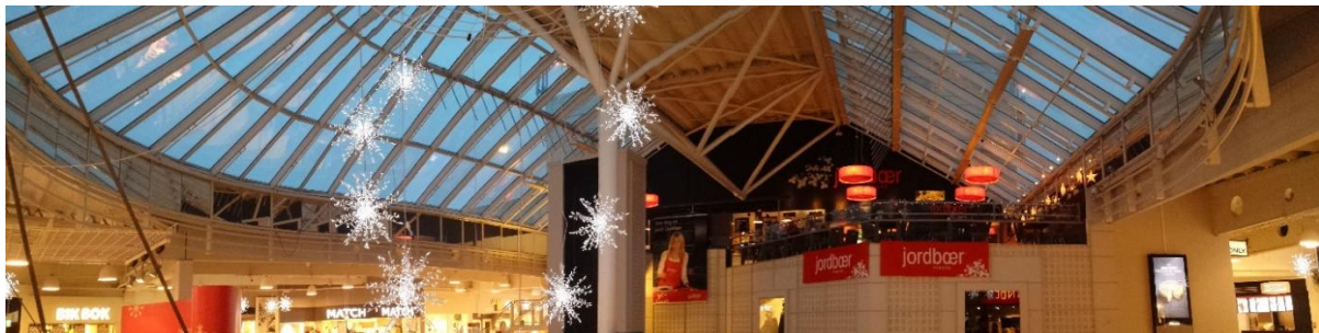
Figure 5-1. Skylights in the central atrium and the cafeteria located on the mezzanine below. Openable windows are present on both sides.
