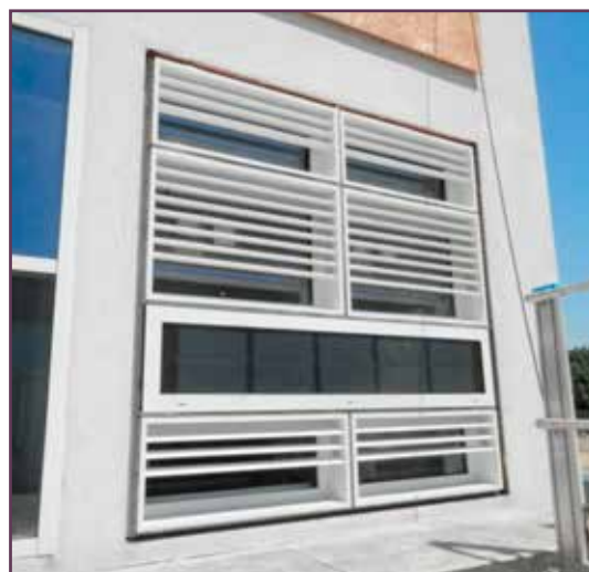
Figure 9.3 - Multifunctional façade energy prototype installed into the laboratory building of ACCIONA in Sevilla (Spain) (left), façade prototype system with the motors installed and connected under monitoring (right). Source: Acciona Construction, R&D Department.
