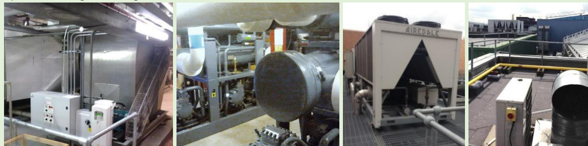
Examples of retrofitting of HVAC installations in two existing centres (Photo: SINTEF Byggforsk)
