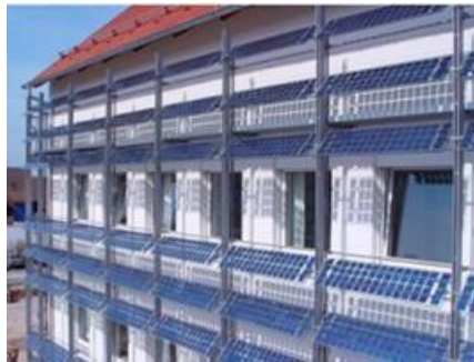
Figure 49: PV panels integrated in external solar shading (Source: http://www.solarpv.co.uk/solar-pv-louvres.html )
