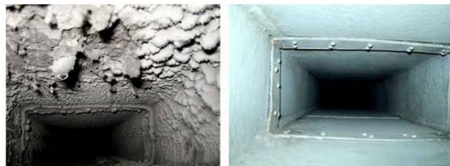
Figure 61 – mould and fungi problem in air duct (Photo courtesy of Clean Middle East Magazine)
