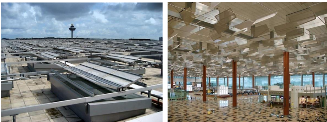
Figure 45 – Example for a specialized roof daylight system: Changi Airport in Singapore, Development by Bartenbach and DURLUM
