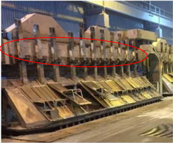
Figure 1: Gas channels at the top of the super structure.
