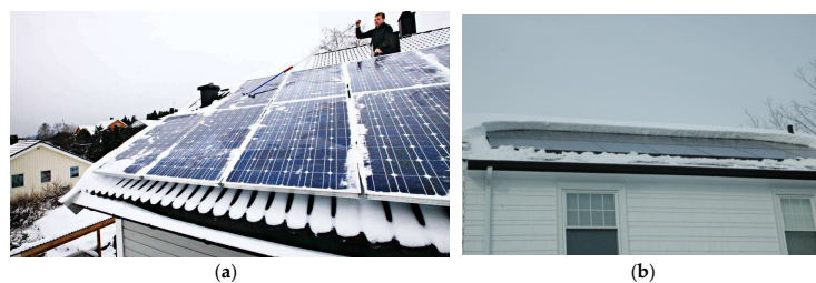
Figure 24. Today, one often has to use manual and mechanical methods for removing snow from solar cell roofs as depicted in the (a) [175] and (b) [176] photos.
