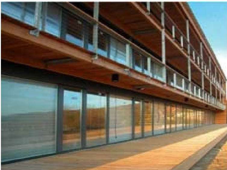
Figure 12 Zero energy office building from Kempen, Switzerland (Cosella-Dörken [23]).
