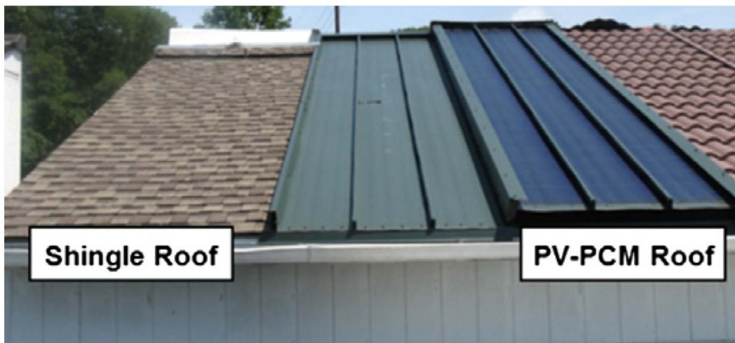
Figure 10 PV-PCM roof (Kosny et al. [62]).
