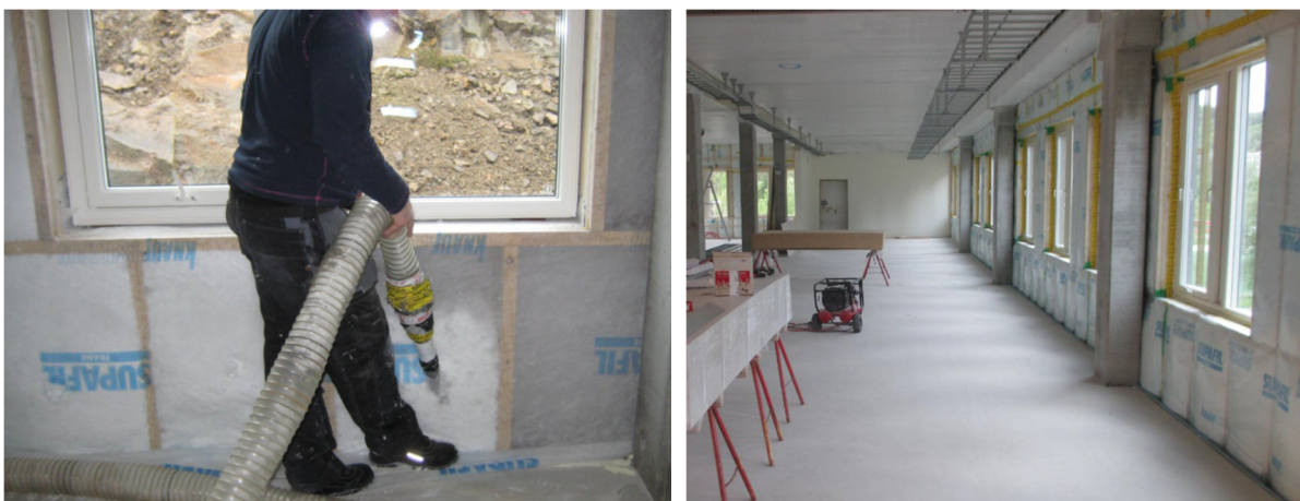
Figure 7.2 Thermal insulation on external walls. Photo: Forsvarsbygg.
