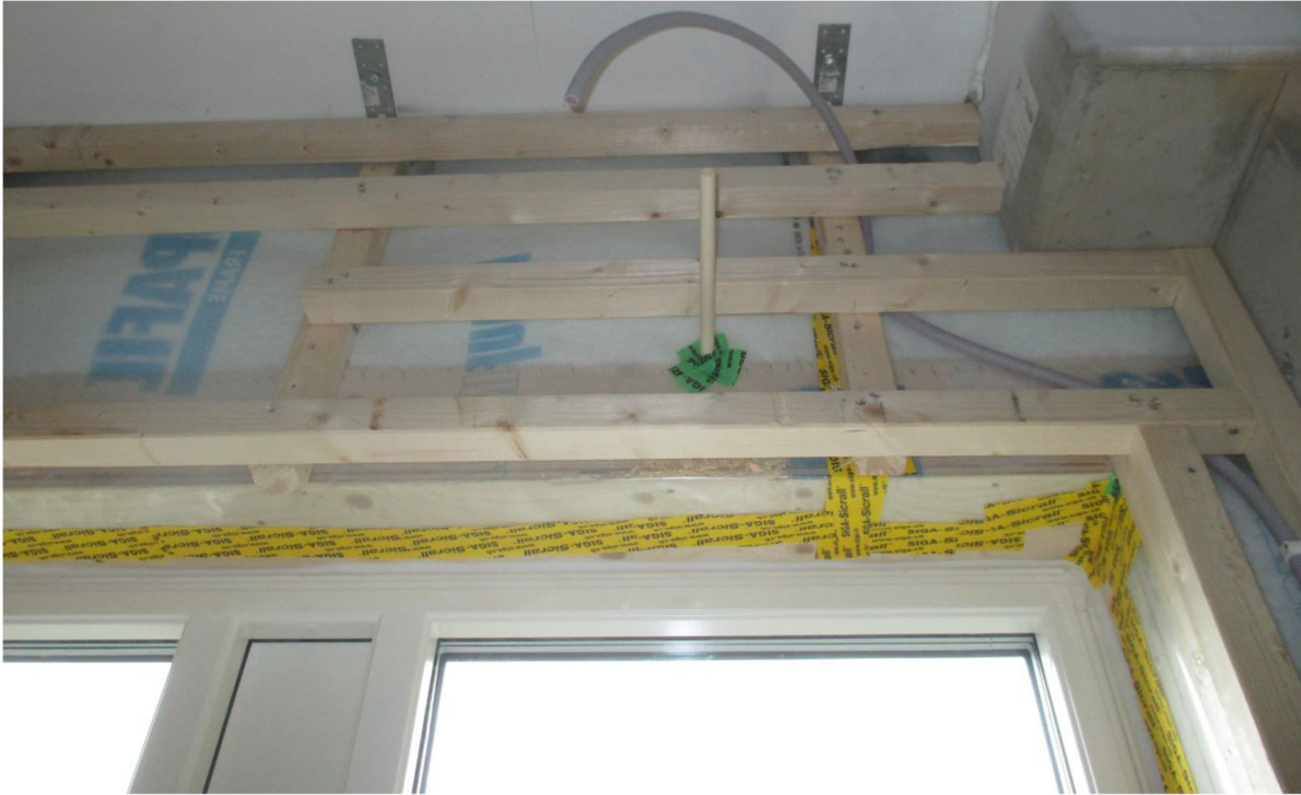
Figure 7.3 Building of air tight walls. Photo: Forsvarsbygg.
