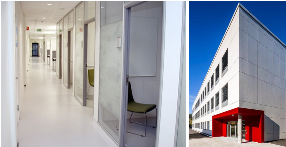
Figure 2.1 Left: Offices in Visund. Photo: Å. V. Sjørusen, Forsvarsbygg. Right: The entrance of the Visund office building. Photo: Forsvarsbygg / Hundven-Clements Photography.
