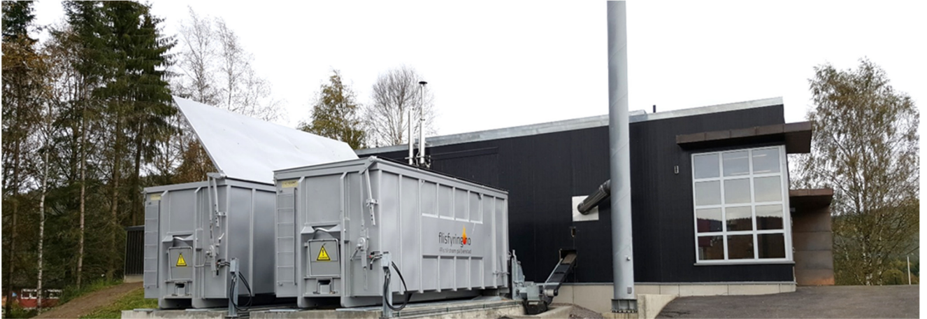
Figure 5.3 Storage silos for the CHP unit at Campus Evenstad, courtesy of ETA Norge AS.
