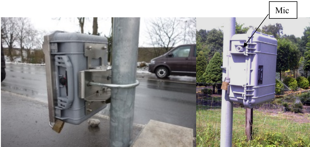
Figure 1: TOPO.Bigbox mounted by the road side (photo left: Torgeir Vaa, SVV, right: RTB)
